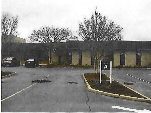
Sign Type B1 / Parking Lot ID Location P.09 (Side B - Same as A)
