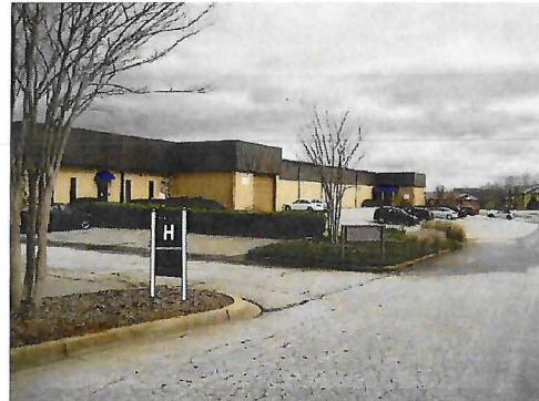
Sign Type B2 / Parking Lot ID Location P.14 (Side A - Same as B)
